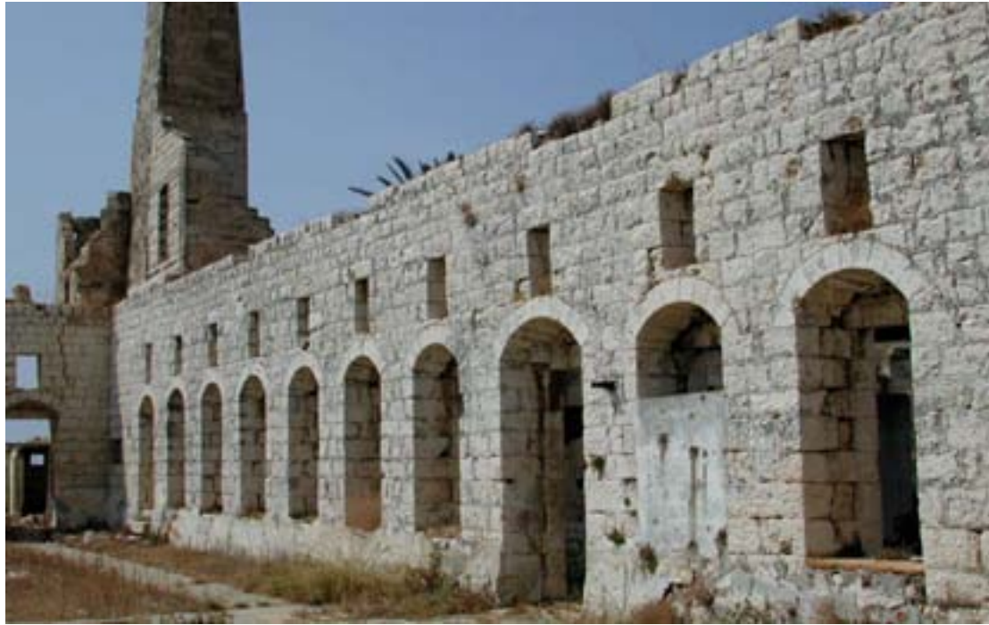
Photo 11 Remains of Silk Factory at Damour. The building maintains the links with the town's important industrial past.
